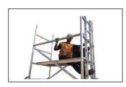
**Step 10** Sitting through the trapdoor add two horizontal braces on 5<sup>th</sup> & 6<sup>th</sup> rung ,two each on both end of the frame.
