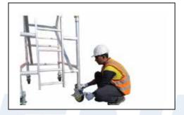
Step 8 Check with the spirit level on both length and width, side of the tower, adjust the wheel if it is required to level the tower.
