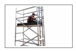
Step 13 Fit the toe board .Slide the side board into the correct slot in the board. Ensuring the object shouldn't fall and trap door opens fully.
