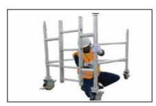
Step 3 Add two horizontal braces, BLUE colour coded, to the vertical member of the frame, as low as possible. All horizontal Brace must fit from inside the tower facing out.
