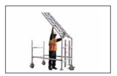
**Step 4** Add further frames ensuring the ladder frames are in line.
