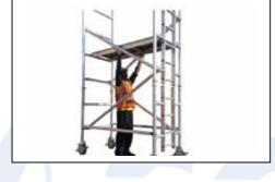
Step 7 Position trapdoor platform on 3rd rungs from the top Make sure the trapdoor opens to the ladder side. Engage windlock. (AS ILLUSTRATION 3)
