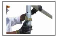
**Step 5**Engage Snap pins to the frames (As Illustration 2)
