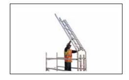
**Step 11** Continue to build the tower using the 3T method as step 4,5,6, 7,10. Till the desired height is achieved.
