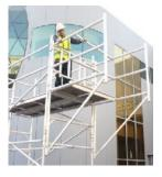
4. From behind the rungs fit an additional set of guardrails to the top 2 rungs on the Cantilever frames.(for single width go to step7) for the new platform, pushing down to lock on
