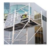
5. Going through the rungs or gate, from behind the new guardrails fit a platform next to the one you are on.
