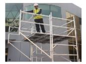
6. Reposition the inner braces to the verticals above the top 2 rungs on the cantilever frames to complete your working guardrails. (Single width cantilever go to step 8)
