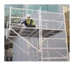
7. From behind the inner set of guardrails fit a platform next to the one you are on.
