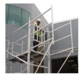
2. Fit cantilever frames; ensure the 3. From behind the rungs line up to avoid trip hazards on the platform decks. Ensure couplers are tight. Repeat on the opposite side.
