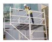
5. Fit an additional set of guardrails to the top 2 rungs on the cantilever frames for the new platform, pushing down to lock on.
