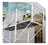
7. Fit toe boards to complete the structure
