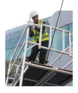
1. Fit 3 Swivel couplers to the vertical above the top rung, below the platform and 2 rungs below the platform. Repeat on the opposite side.
