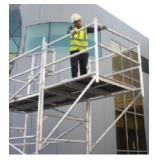
6. Reposition the inner set of braces (Double width Cantilever only)
